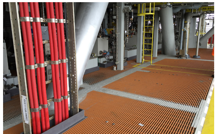
Phenolic grating installed on an offshore platform in the North Sea. Photo courtesy of NOV Fiber Glass Systems
